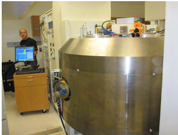
Target carousel filled with targets. Left side of cyclotron has electrical power panels and target support units.
