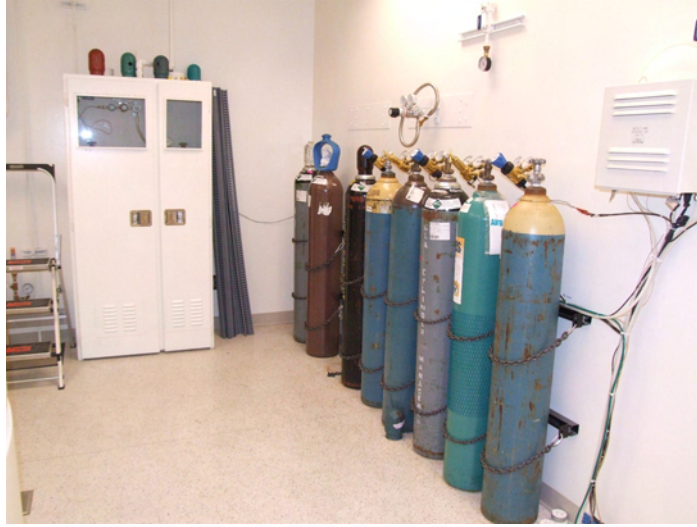
Gas tanks used for cyclotron operations. Hydrogen is explosive at almost any concentration, so it is housed in a separate ventilated enclosure.
