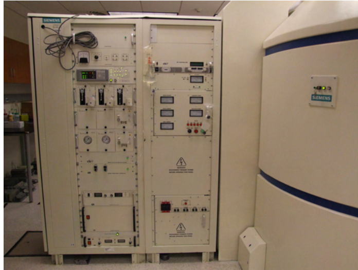
Power supply cabinets for cyclotron, also includes target support units.
